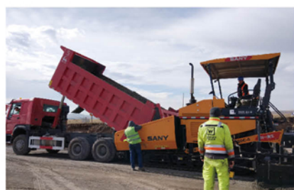
碎石基层摊铺 Paving of macadam base
