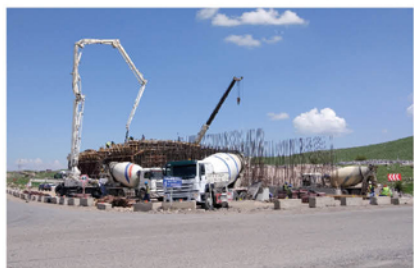
大型农业通道施工 Construction of large agricultural passages
